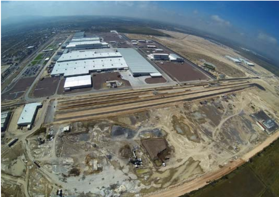
HOT SPOT A recently completed auto assembly facility for Nissan in Mexico, which has plans to expand.
