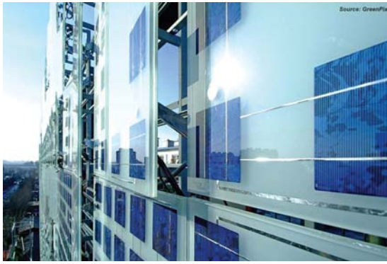
The Zero Energy Media Wall – harvests solar energy by day and uses it to illuminate the screen after dark is an example of sustainability solutions in Chinese cities
