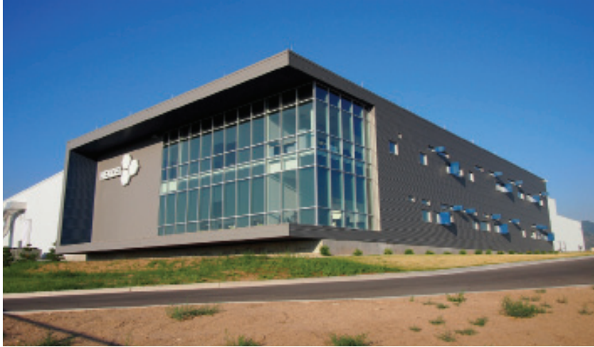
HOT MARKET Hexcel is allocating capital to expand its carbon fiber manufacturing plant in Utah.
