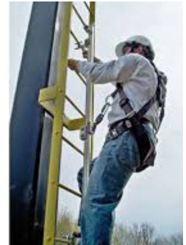
Ladder fall arrest system.
